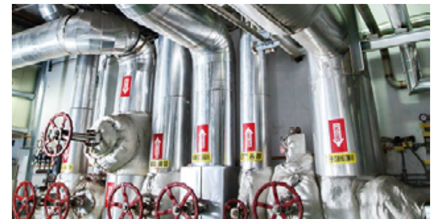
Steam pipelines for recycling external waste heat
